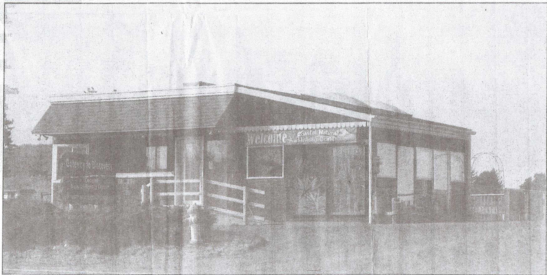
LORI ASSA — The Daily Astorian The Gateway to Discovery in Seaside will be the home of the Wilbur Ternyik statue. The statue was commissioned by The Bridges Foundation of Turner.
